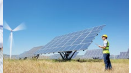
Power generation see pages 62–63
