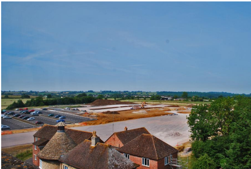
New Mills development in progress
