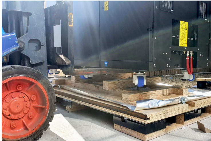
Figure 63 Lifting the system clear of the base of the crate
