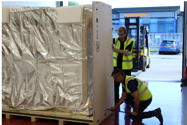
Figure 55 Supporting and removing end panel clips
