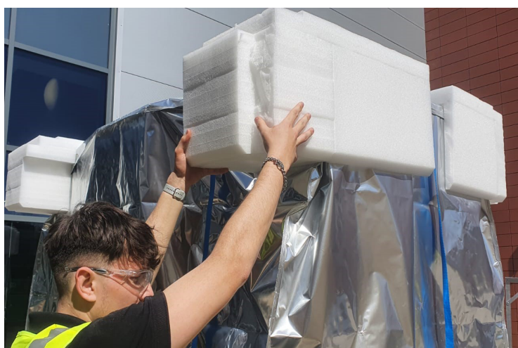
Figure 58 Remove the foam corner packing pieces
