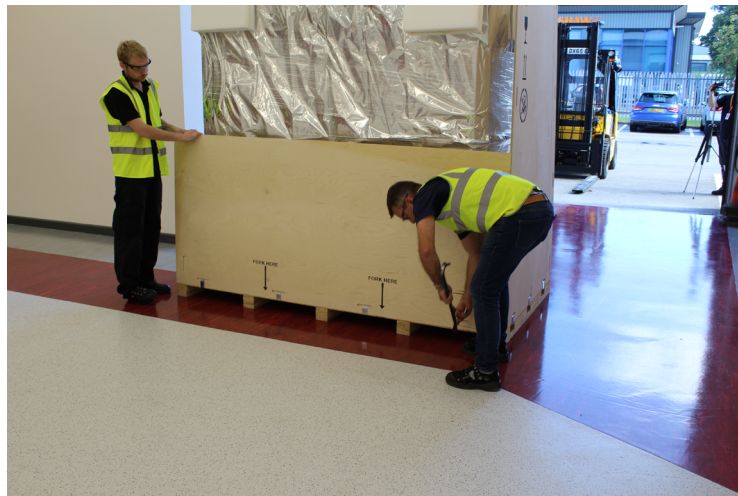
Figure 53 Supporting and removing back lower panel clips
